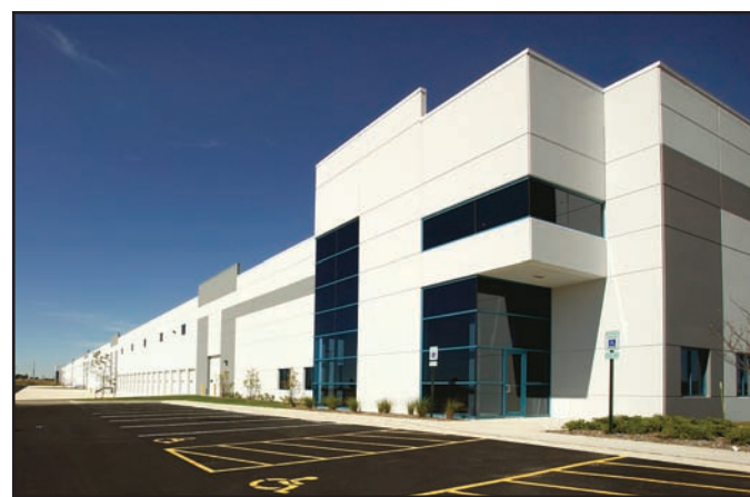
Del Monte Corp. signed for 364,755 square feet this year at LogistiCenter at Rochelle, a DP Partners development.
